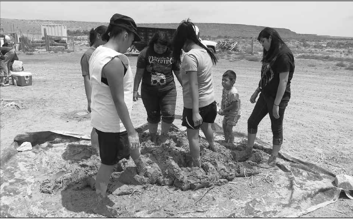
Members of the youth programs use their feet to mix mud and straw to make mud balls that will be use to build the bread oven.
