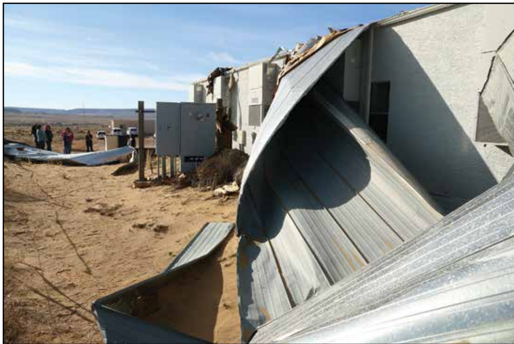
The sheet metal layer of the Kykotsmovi DES Office roof was blown off by heavy winds that peaked at 67 mph on Sunday.
