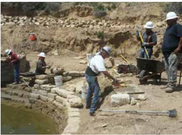
Installation of retaining wall around pond pictured from left to right: Steven Honanie, Lamual Howato, Leon Lalo, Lindsey Koinva and Albert Silas III.
