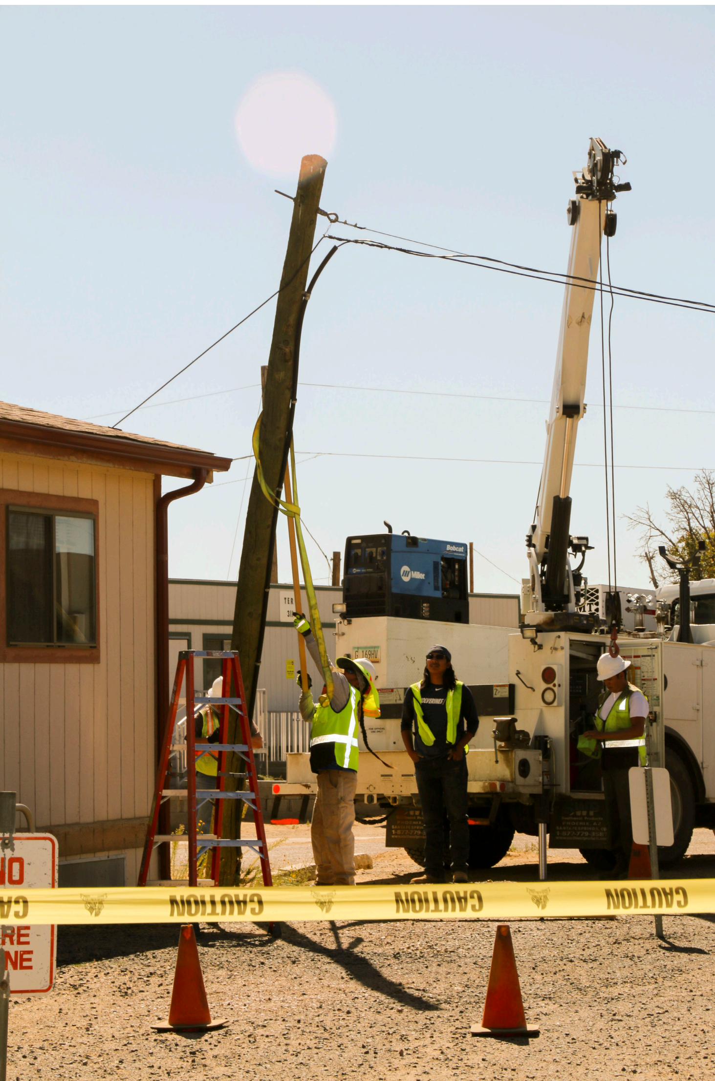
Utility pole being hoisted by crew, making sure of everyone's safety (Photo by Romalita Laban/HT)
